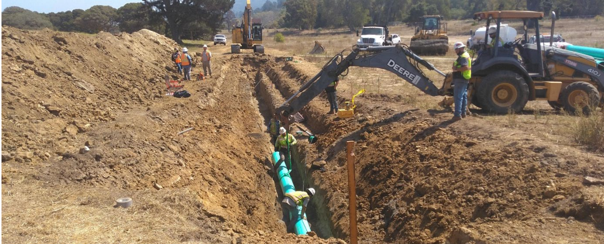
Graniterock Construction Co. installing new 16" sewer line at Palo Corona Park
