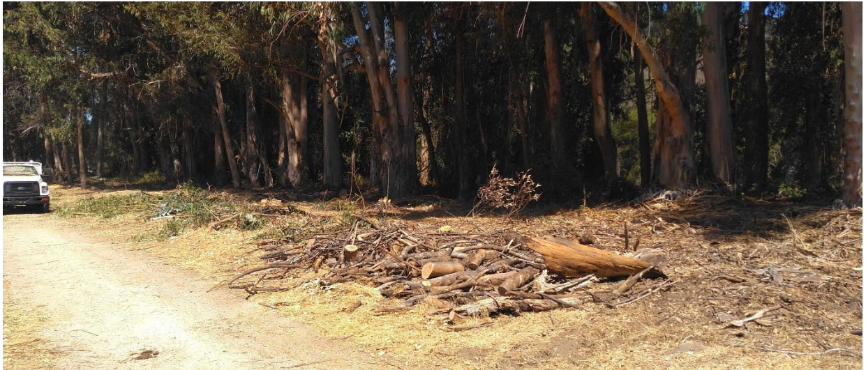
A newly constructed 30' fuel break along the Rancho Loop Trail
