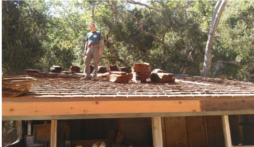
Ranger John working on Kahn Ranch's Goat Barn Roof
