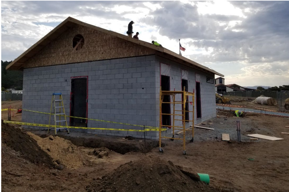
Restroom Building Walls and Roof Framing
