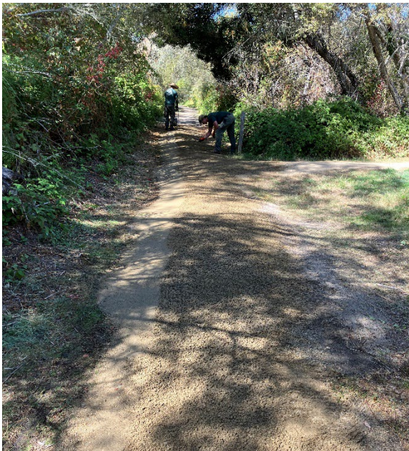
Rangers adding and compacting material at Frog Pond Wetland Preserve
