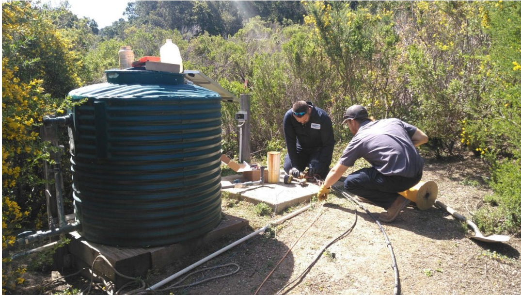
Dougherty's Technicians Working on Mesa Well Pump
