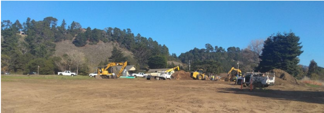
Graniterock finishing pipe installation on RCU east course
