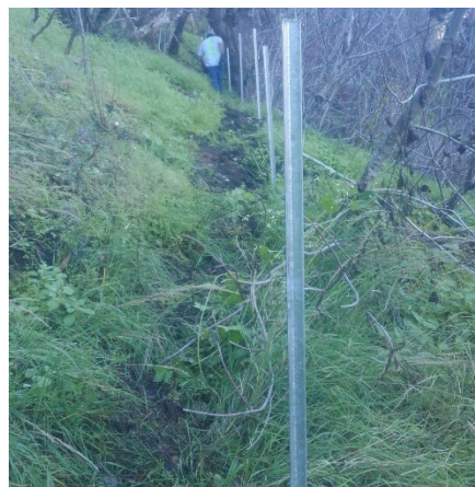
Section of new galvanized t-stakes
