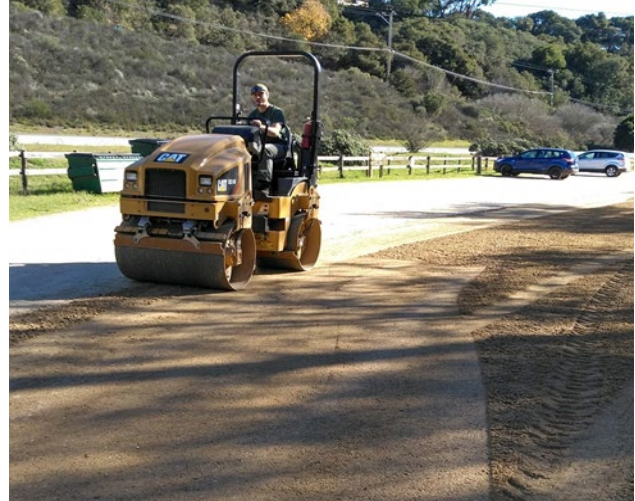
Ranger Hatton rolling/compacting
