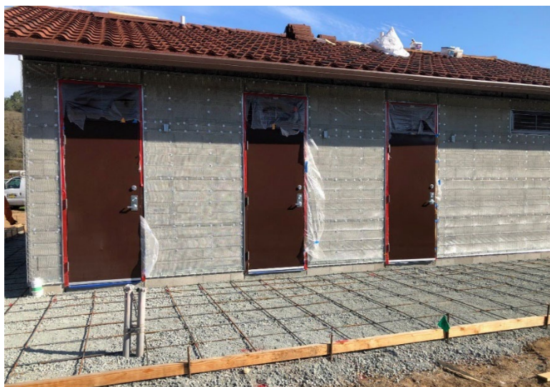
Doors Installed; Walkway Ready for Concrete
