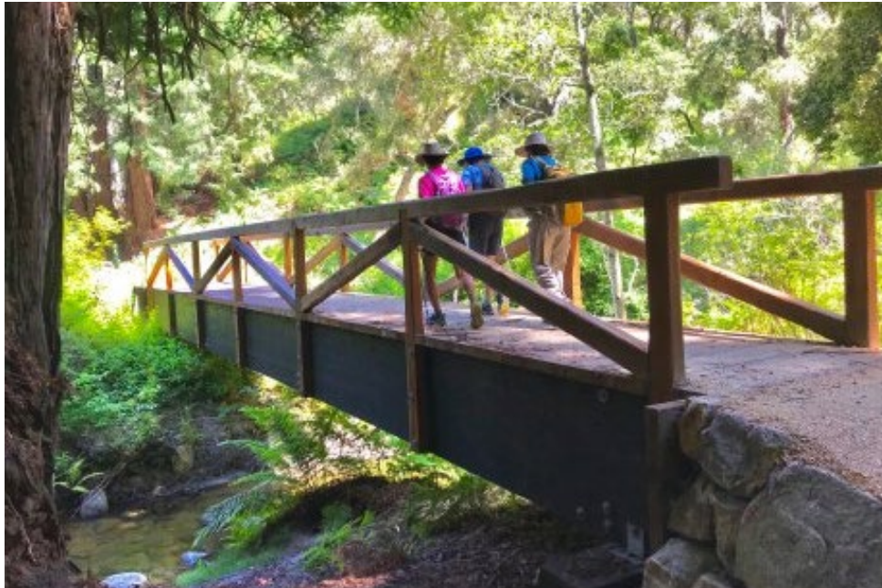
Pedestrian Bridge Spanning San Jose Creek
