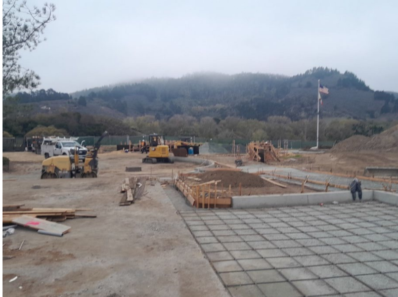
Accessible Parking & Bus Pull-out Being Prepared
