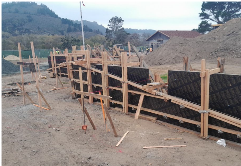
Shade Structure/Bench Retaining Wall's Rough Forming
