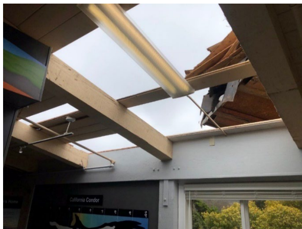
Dry Rot Removal of Discovery Center's Roof Sections
