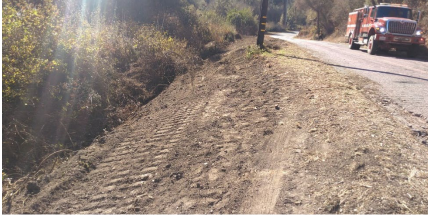
Roadside Fuel Break Prior to Suppression Repair
