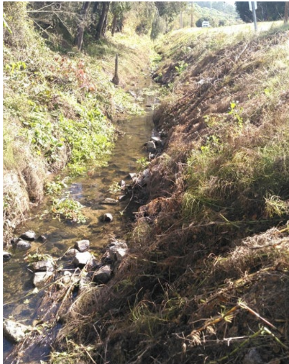
Highway 218 Drainage Canal
