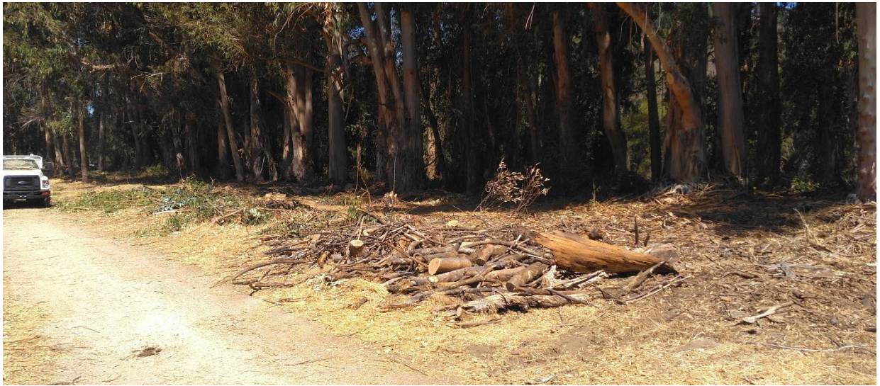
A newly constructed 30' fuel break along the Rancho Loop Trail
