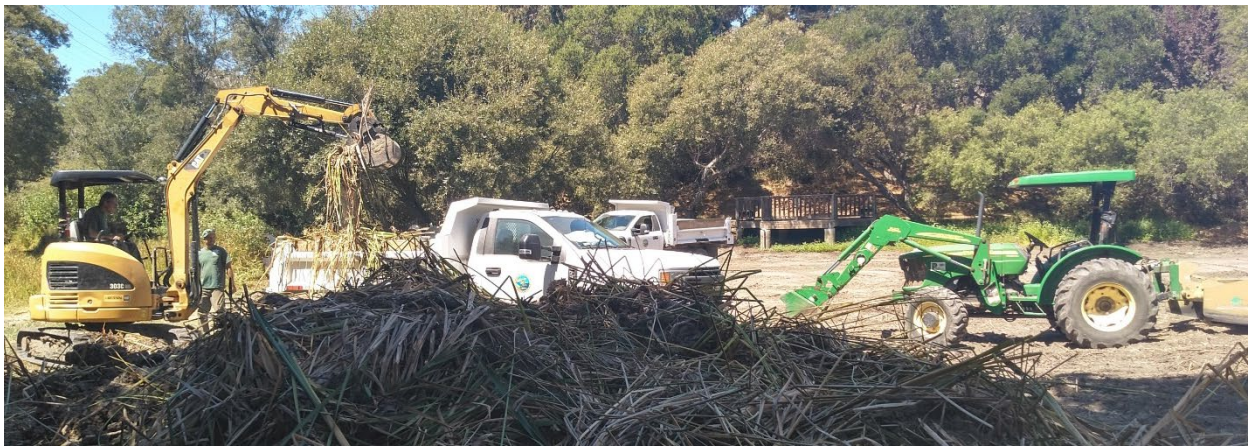
Ranger John loading excavated tullies into District dumptrucks
