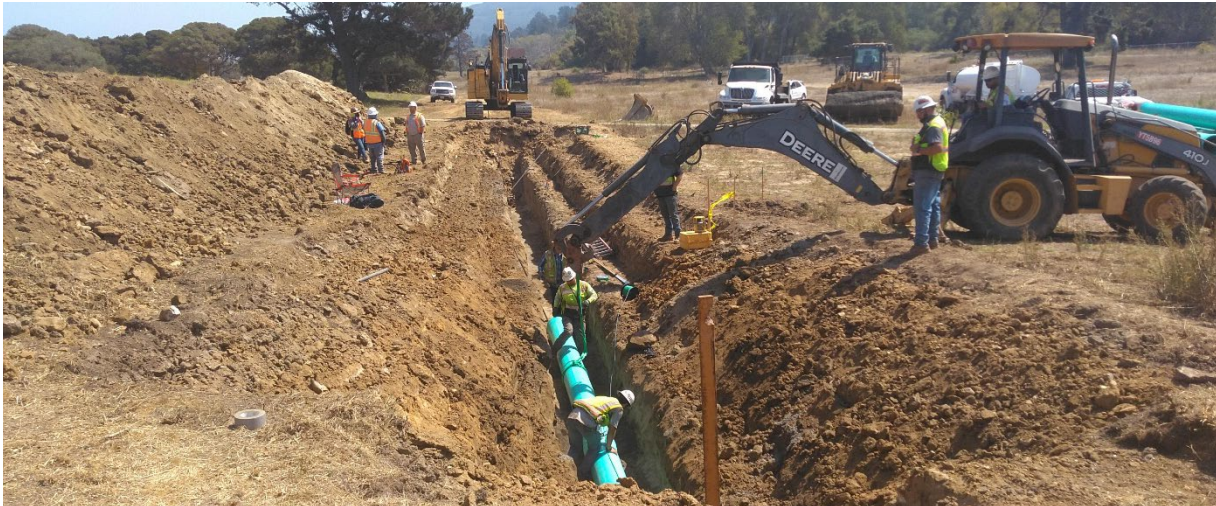
Graniterock Construction Co. trenching and installing new 16" sewer line
