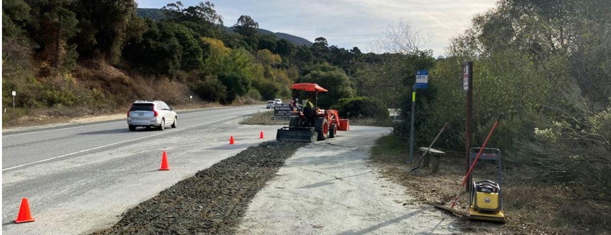
MPRPD staff and equipment “ripping” entrance ramp
