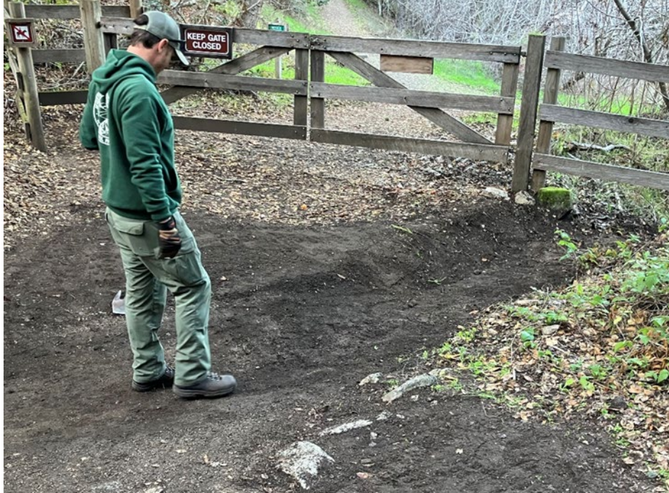
Maple Canyon Trail drain dip cleared and compacted
