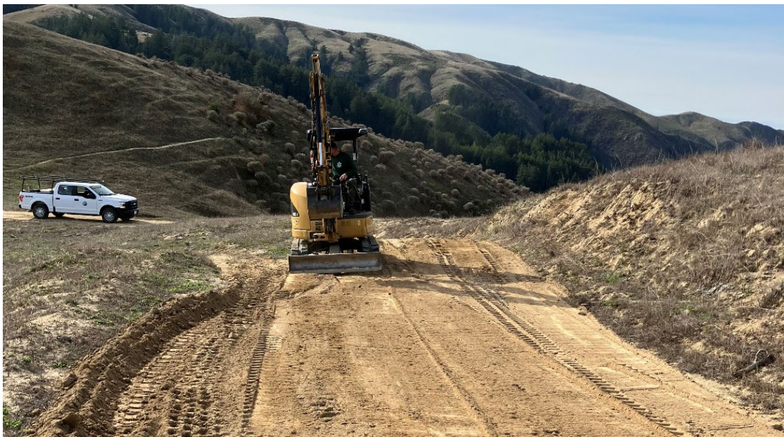
District excavator clearing dips in PCRP backcountry
