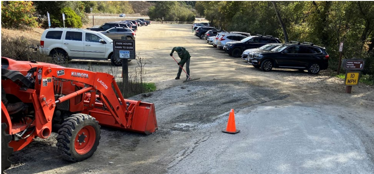
Prepping for compaction at base of entrance ramp
