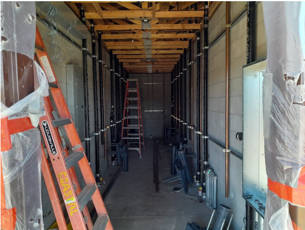
Restroom mechanical chase
