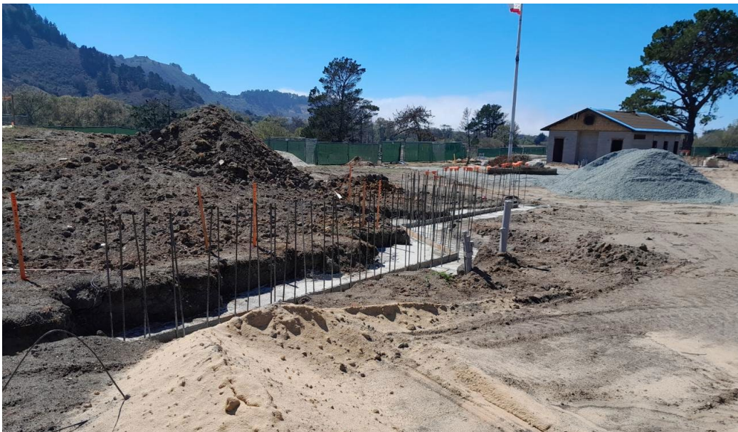
Retaining / Landscape wall footing
