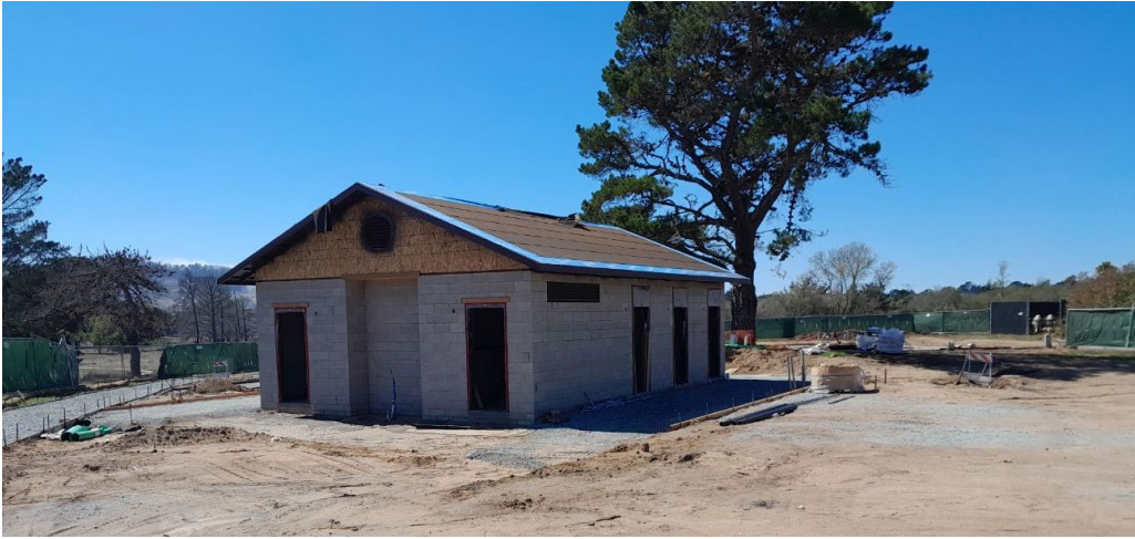
Restroom roof framing and eave paint
