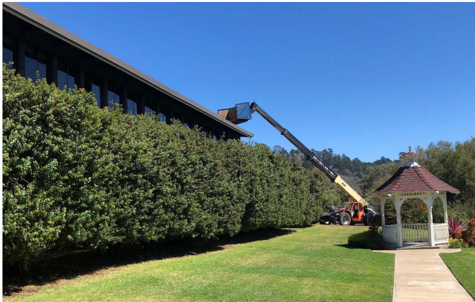
Back side of the Merienda Room
