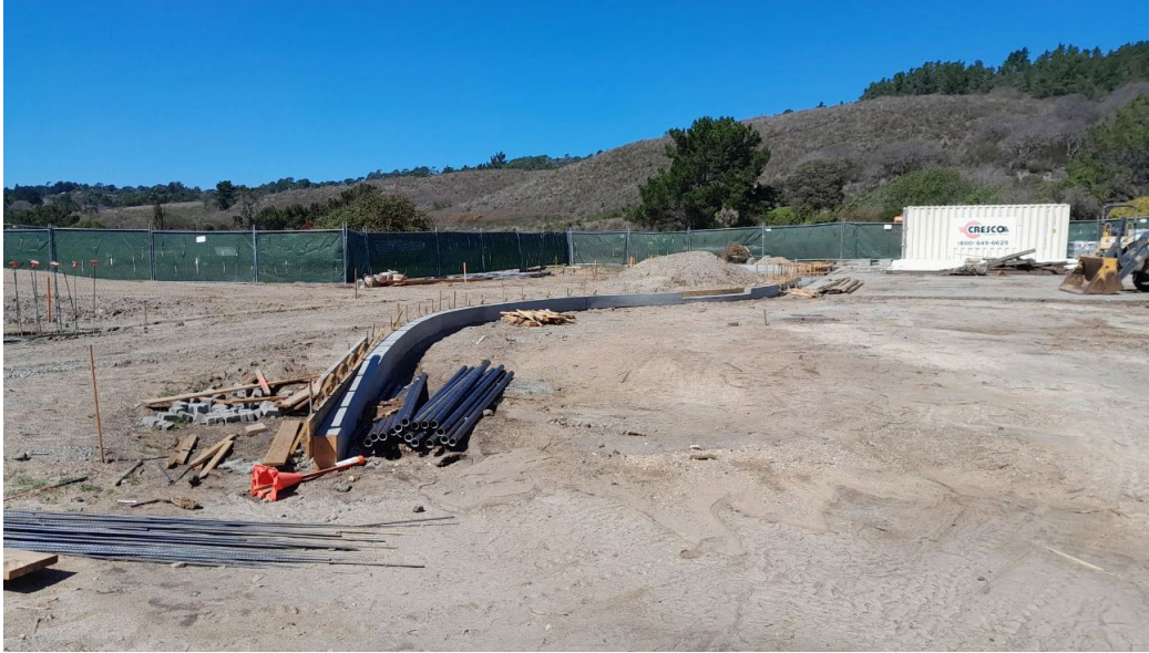
Retaining / Landscape wall footing
