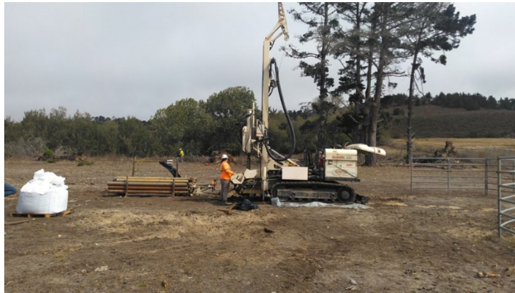
Test Well Drill Rig
