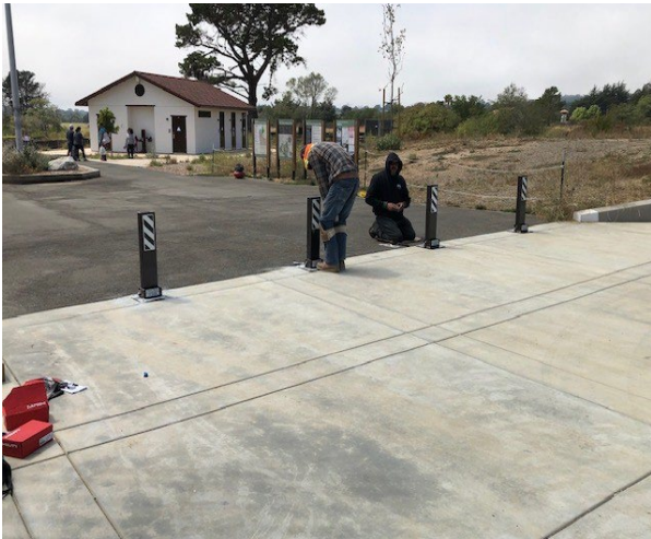
Bollard installation
