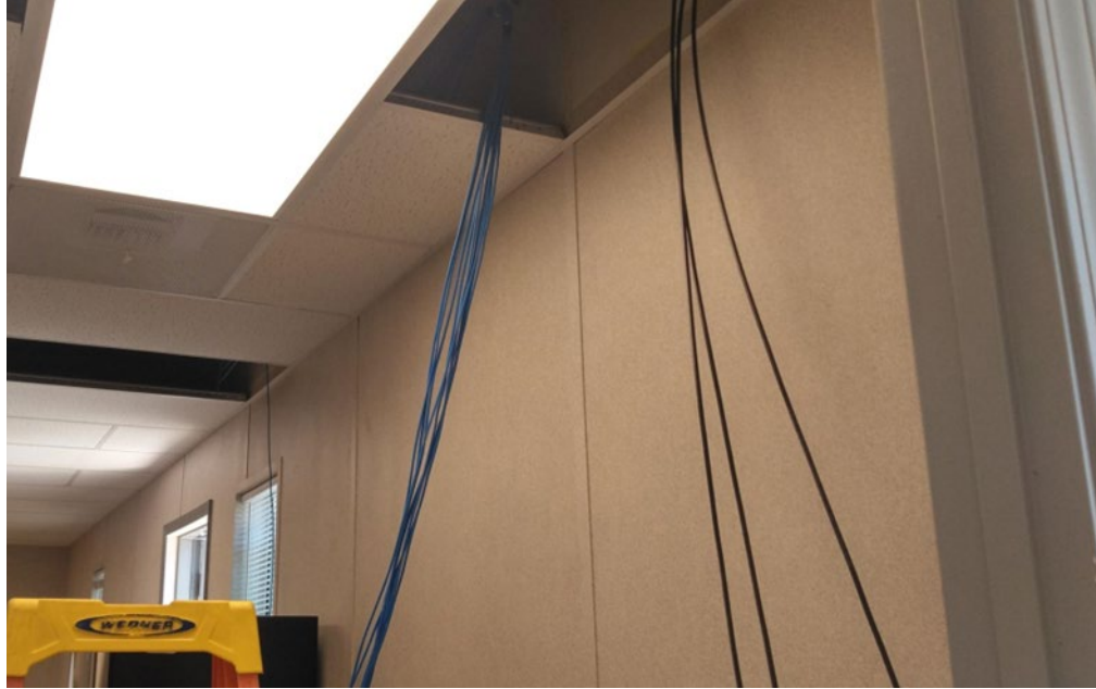
Cables being run throughout the ceiling
