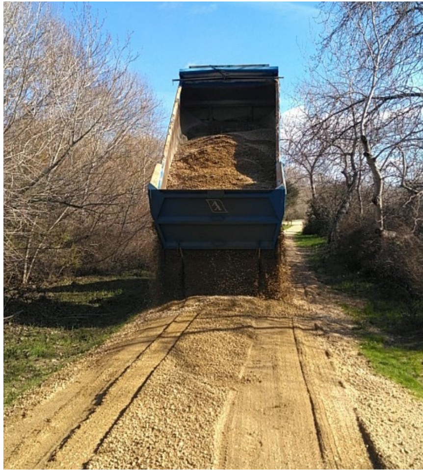
Clean-up and Restoration Begins (continued)
