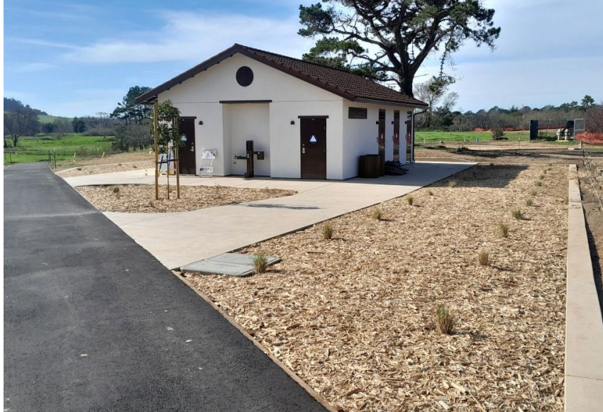
Restroom facility, landscape, and concrete pathway
