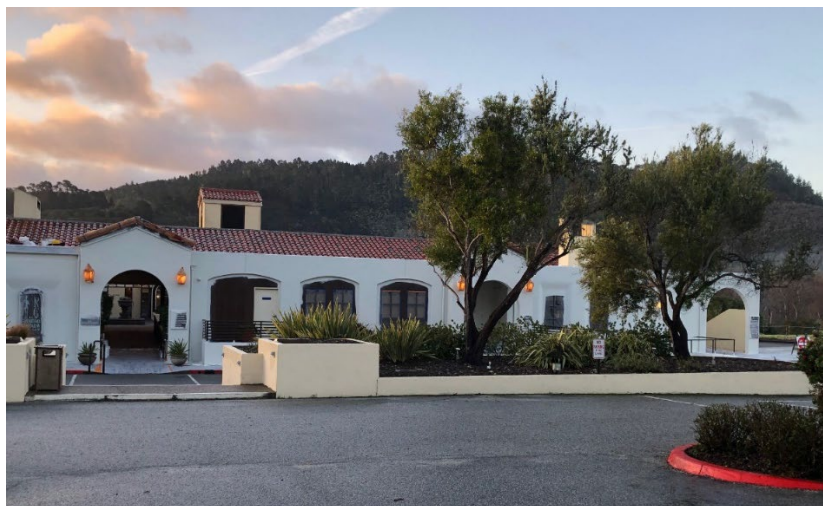
New paint application matching the new restroom building
