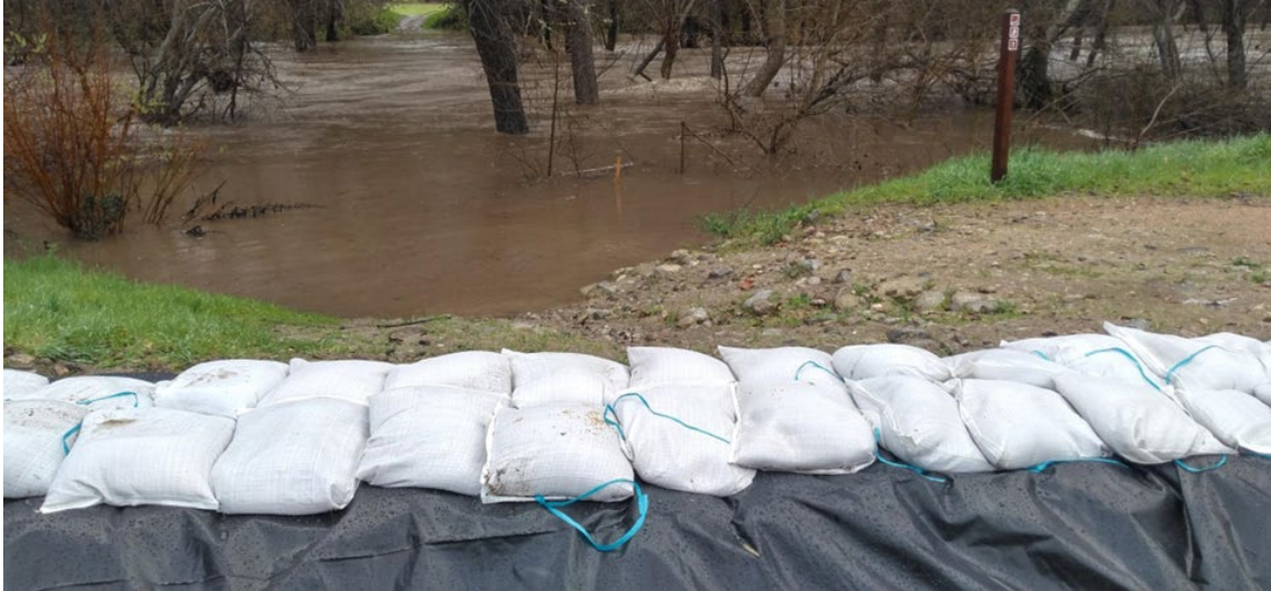
DeDampierre Temporary Sandbag Flood Wall Constructed
