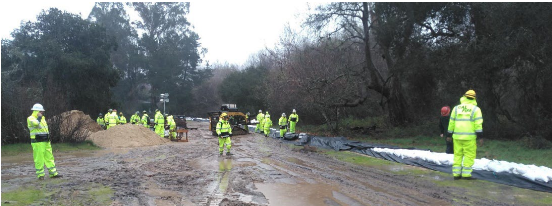
DeDampierre Temporary Sandbag Flood Wall Construction (Middle and Bottom Photographs)
