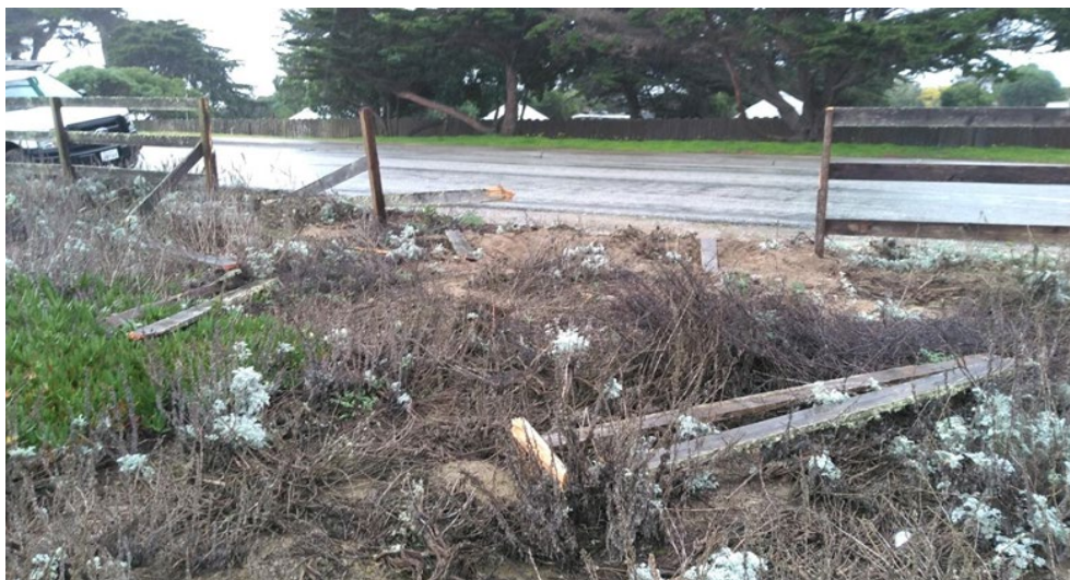
Damaged section of boundary fencing at Marina Dunes Preserve
