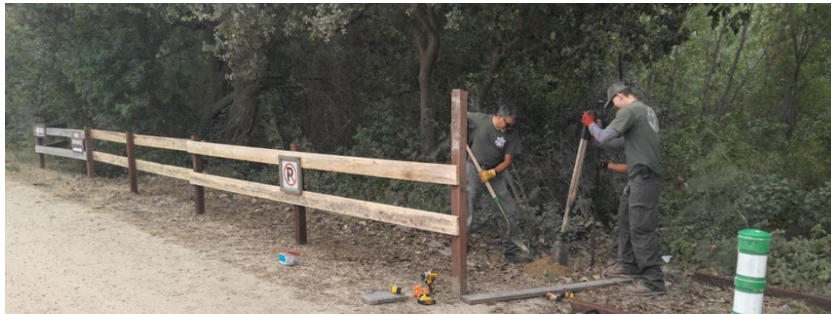
Rangers Joe and Hatton Installing Fencing at GRRP
