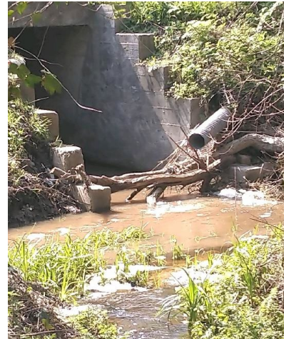
HWY 218 Culvert Inlet
