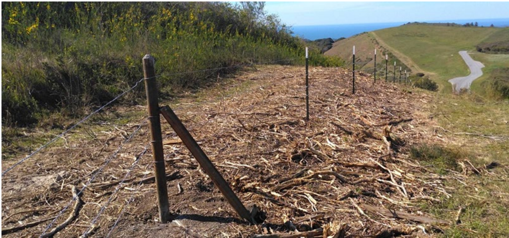
Finished Perimeter Fencing Along MPRPD/SLC Property Boundary
