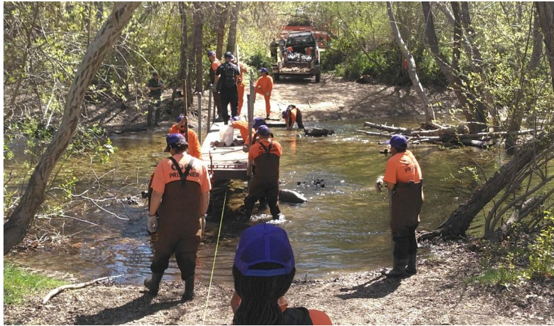
Gabilan Inmate Crew Installing Seasonal Footbridge
