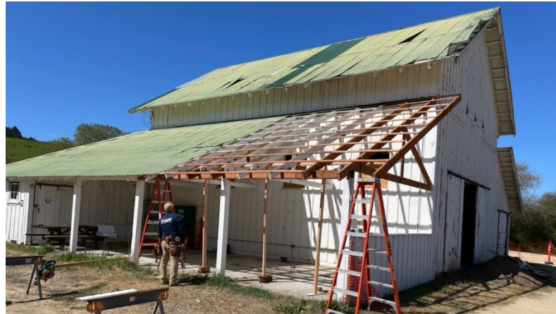
Sharp Engineering Working on Palo Corona Barn Roof
