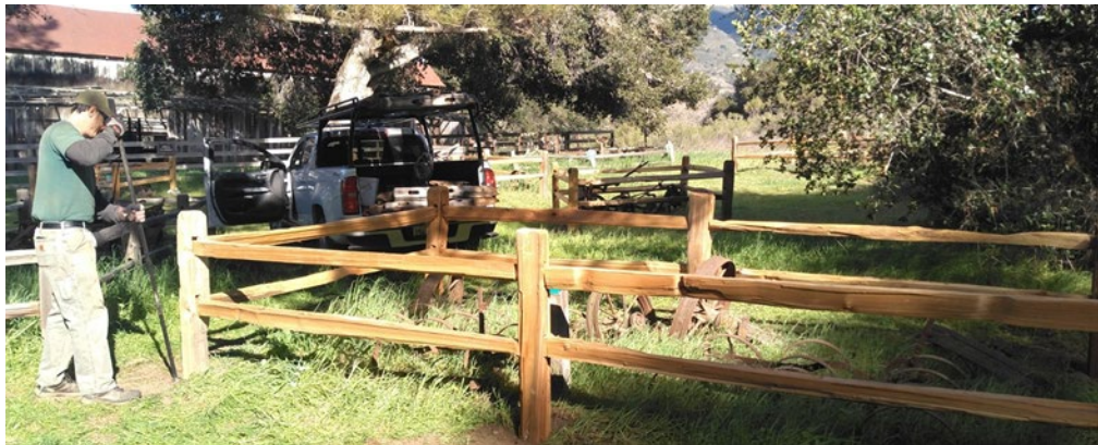
Ranger Vandervort Tamping Split-rail Posts
