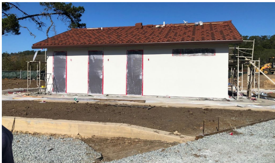
Integrally colored stucco finish coat has been applied
