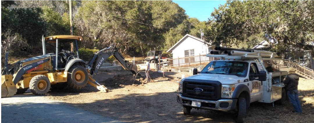
PSTS repairing GRRP Ranger Station septic drain line
