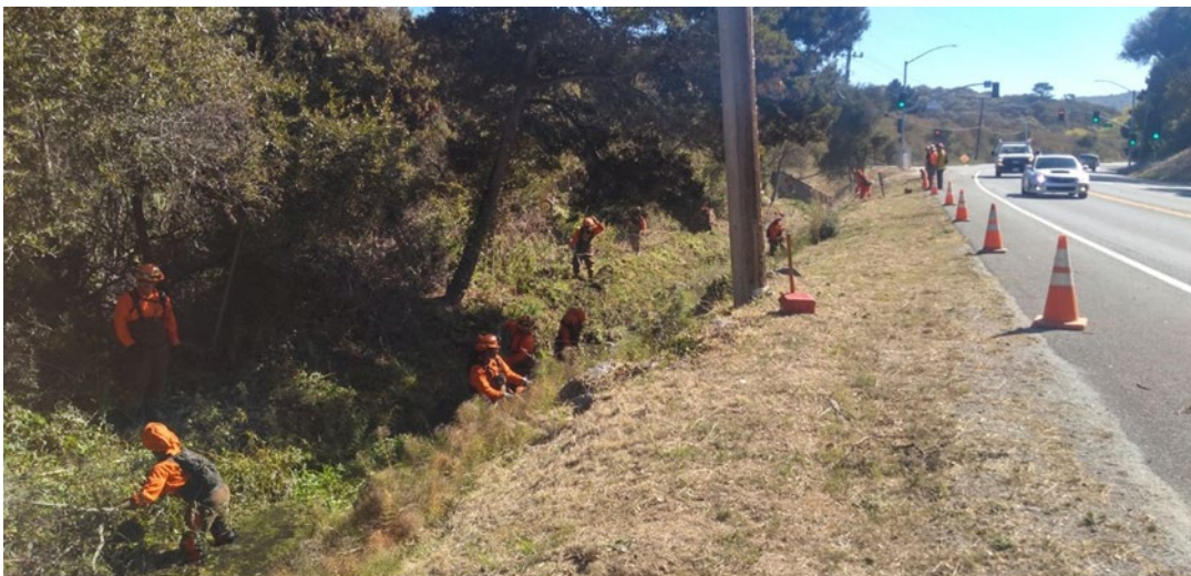
Gabilan Inmate Crew clearing Highway 218 drainage
