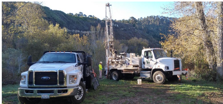
Geo-Con Drill Rig performing core sampling
