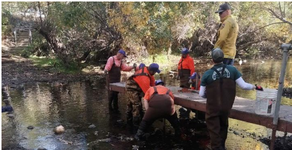
Inmate Crew and Rangers removing seasonal footbridge near GRRP Visitor Center
