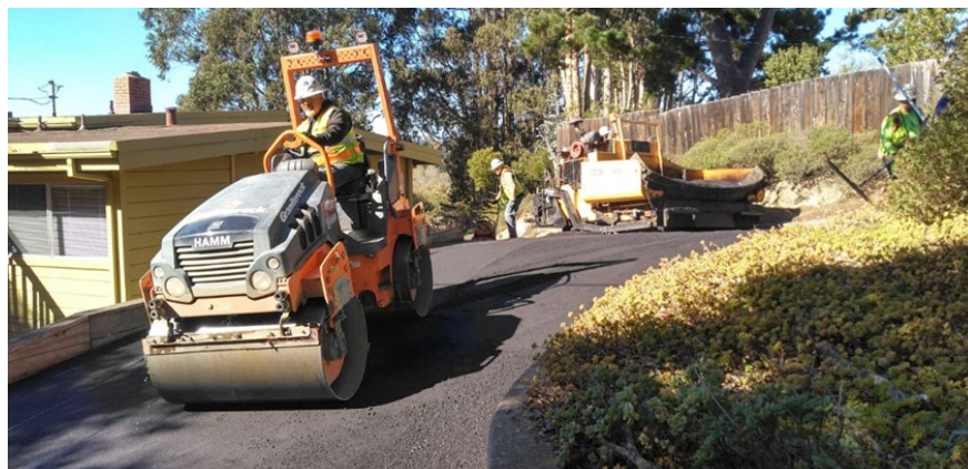
Graniterock roller and paving machine
