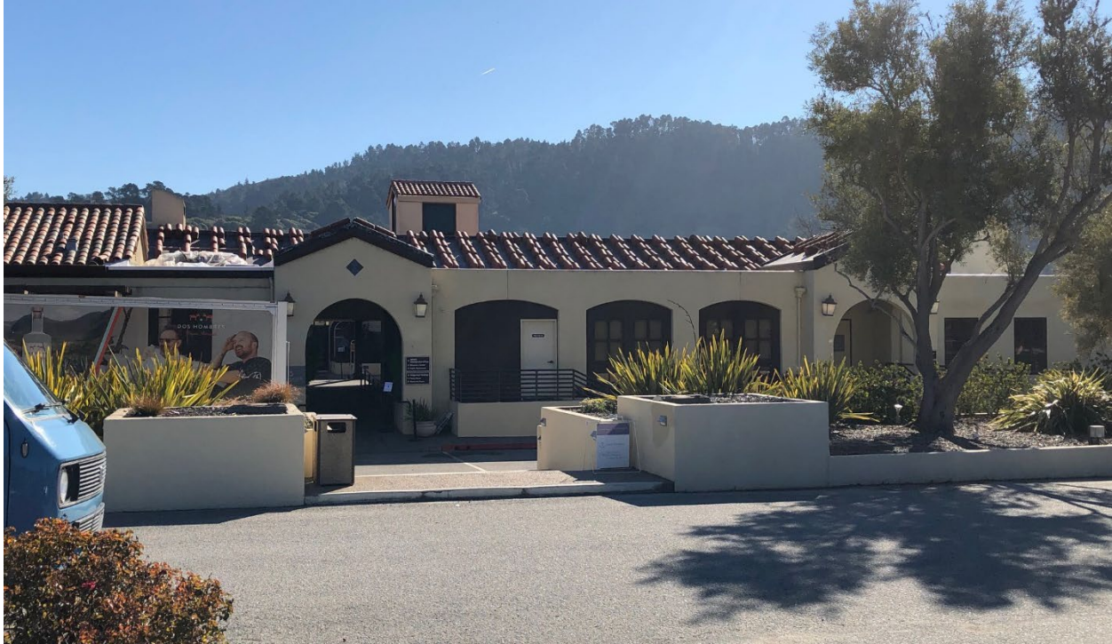
Tile roofing replacement in progress over MPRPD’s administrative offices
