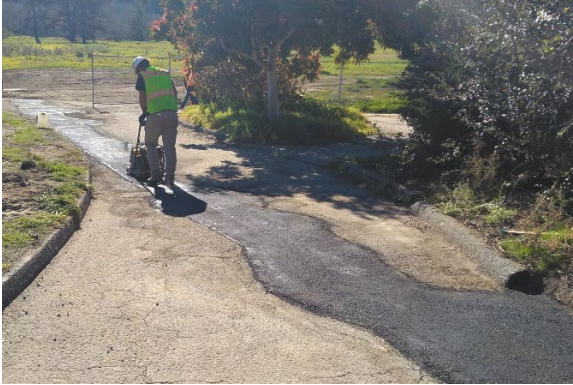
Graniterock Construction Company patching asphalt trails
