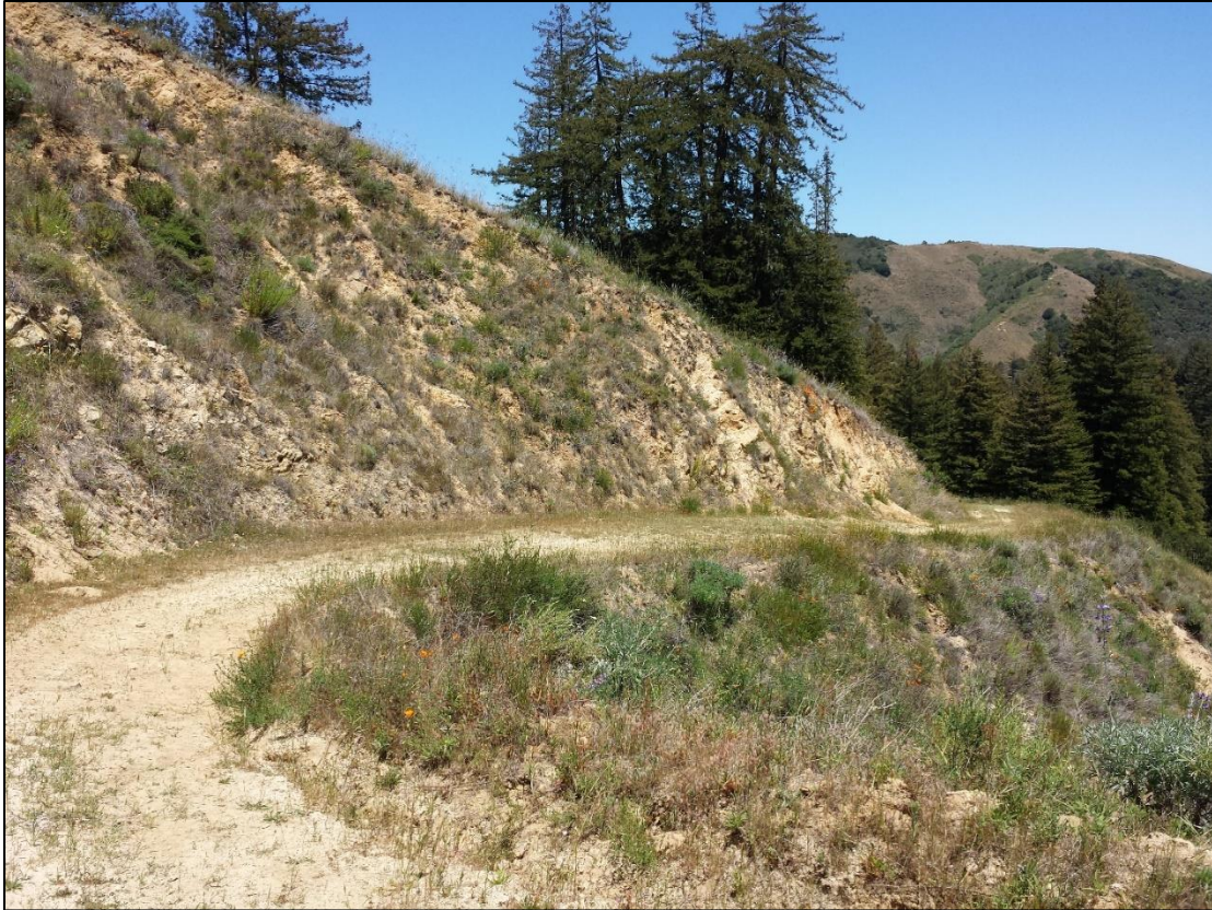
Figure 10 is looking down-hill towards the landslide repair site, which is around the corner just out of view. The roadcut above the ranch road, as well as the slope below the roadbed are vegetated with a mix of Coastal Scrub species, including seacliff buckwheat.
