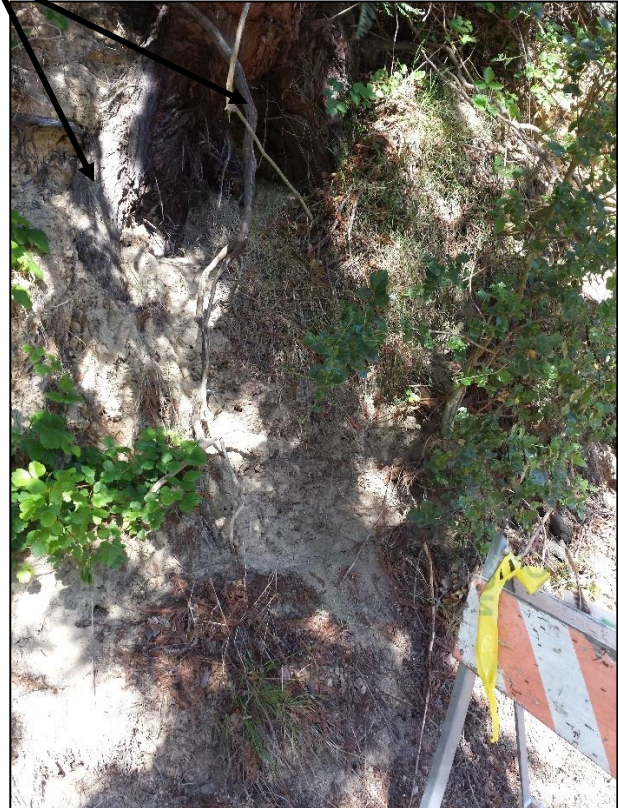
Figure 14 – Exposed redwood roots.
