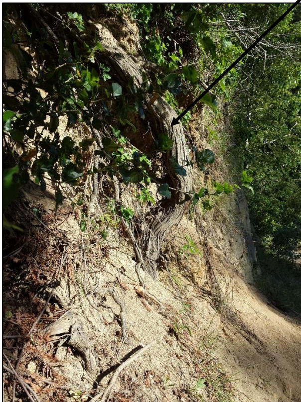
Figure 13 – Exposed redwood roots in the old Roadcut above the apex of the landslide.
