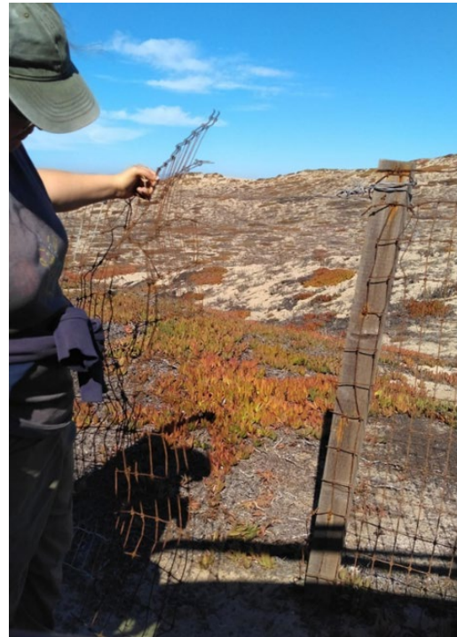
Boundary fence repairs
