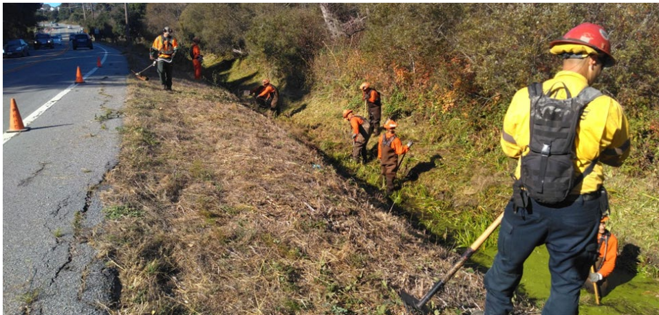
Gabilan Crew clearing FWP drainage channel
