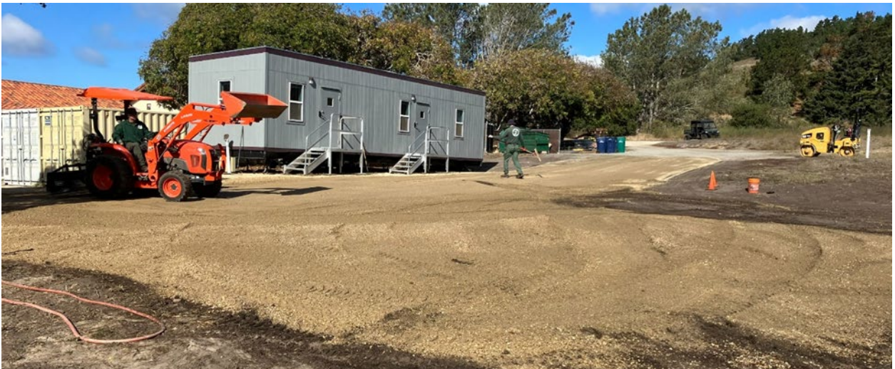
Ranger staff spreading and compacting material using MPRPD equipment
