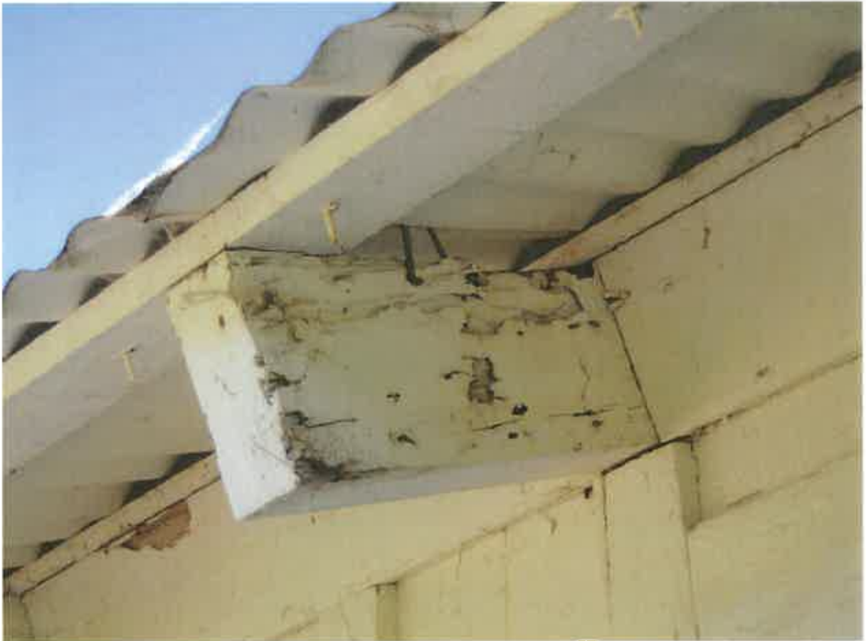
Figure 58. Typical deterioration of roof rafter ends.
