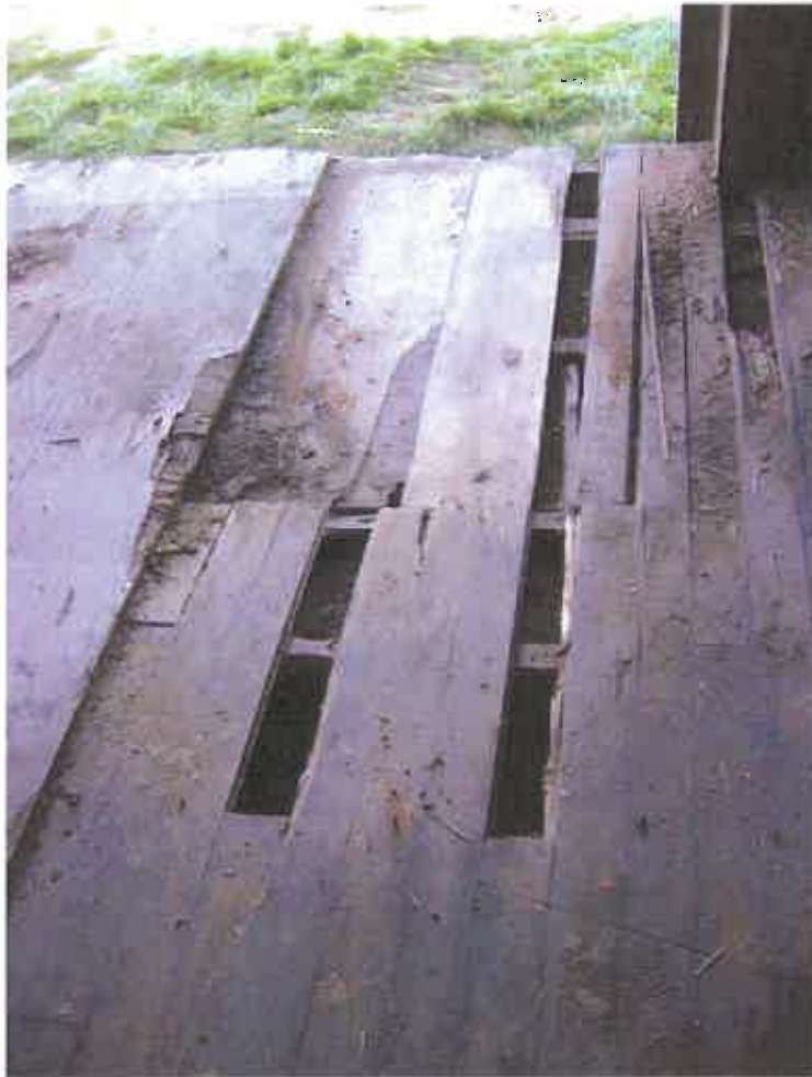
Figure 63. Deteriorated floorboards at the center aisle.
