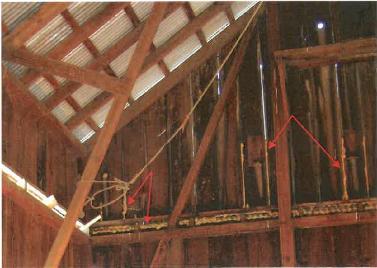
Figure 50. Expandable foam insulation used to fill gaps between exterior siding at the south elevation of the center aisle.
