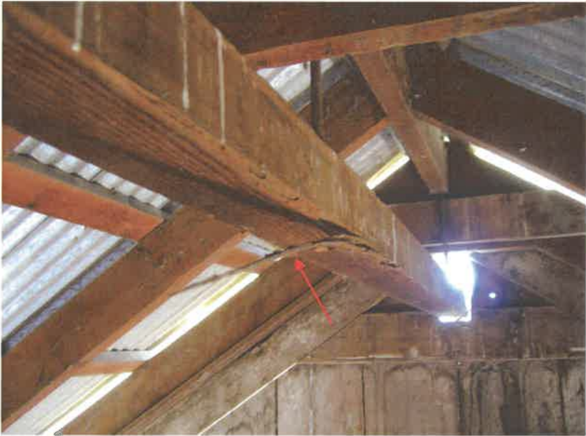
Figure 57. Surface deterioration showing separation of wood fibers at the hoist rail used to move the hay fork.
