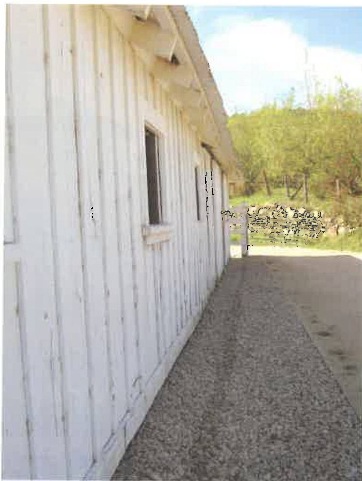
Figure 9. French Drain at the west elevation.
