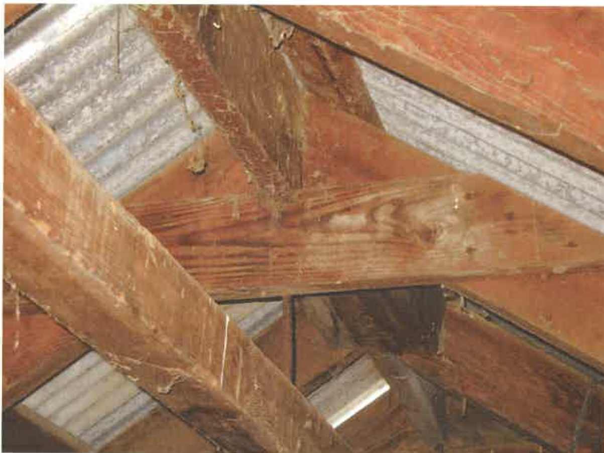
Figure 27. Roof framing system at the center aisle showing where rafters join the ridge beam. Square member below used as a track for the hoist.
