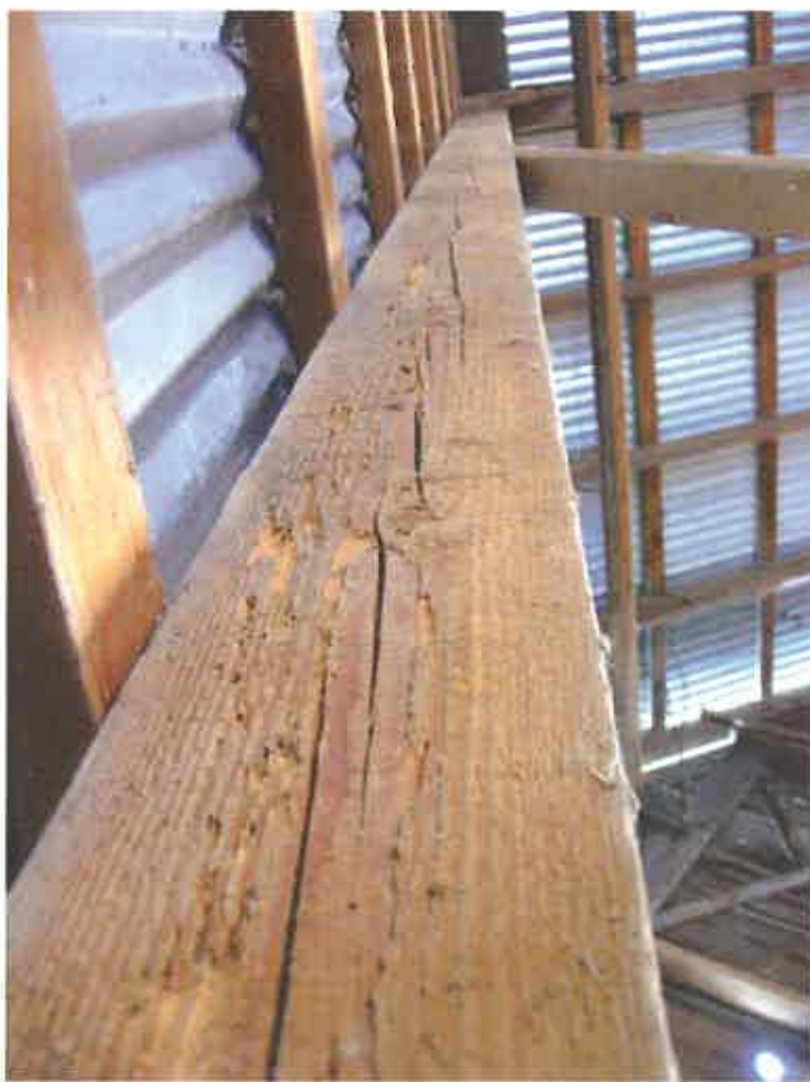
Figure 55. Splits found on timber posts.
