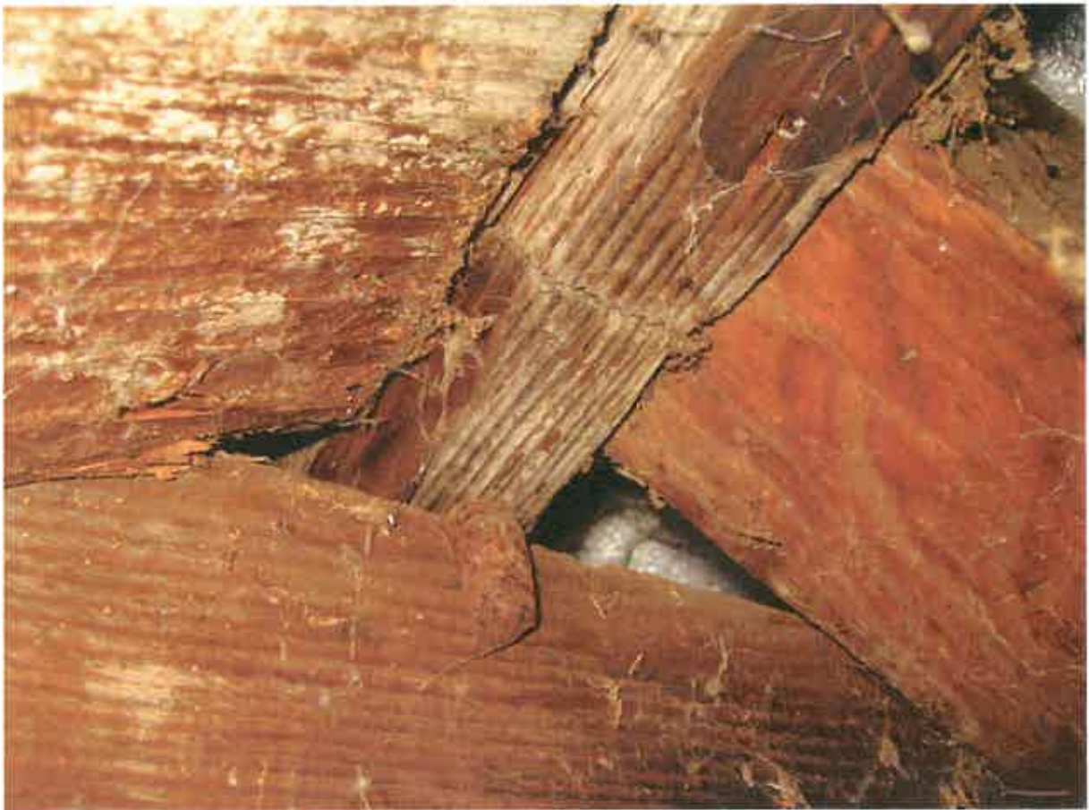
Figure 56. Deterioration at the roof framing system.
