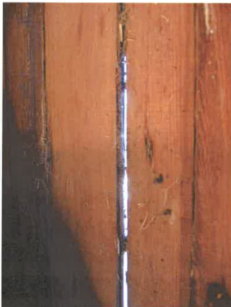
Figure 51. Typical gap between exterior siding.
