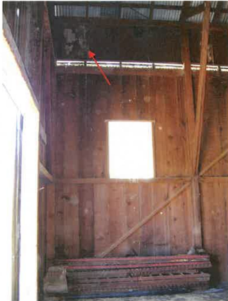
Figure 64. Water stains on the wood boards at the northeast corner of the center aisle. And old rail track stored on the fragile floorboards in the center aisle.
