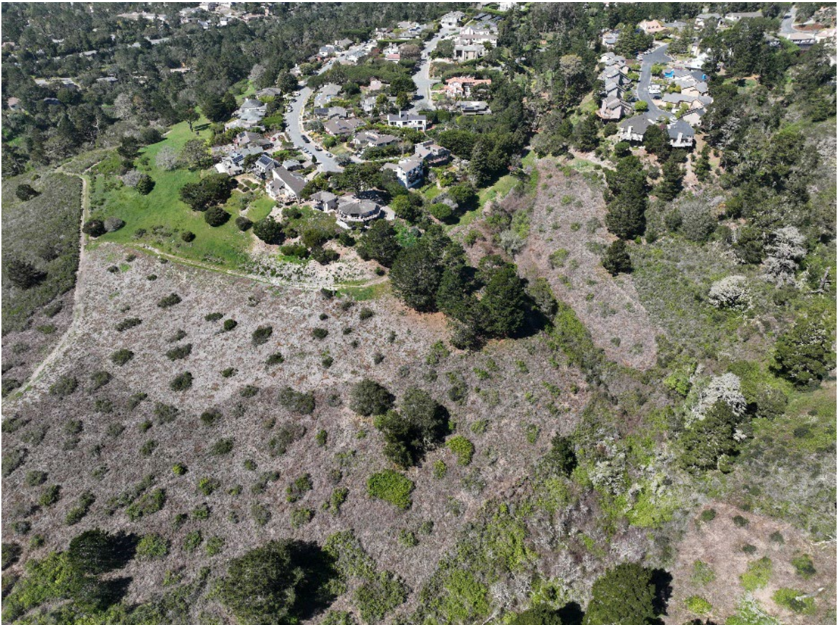
Drone aerial image of the Hatton Canyon Open Space Preserve after RCDMC and District implemented fuels reduction across the property.
