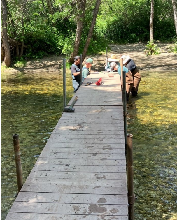
Carmel River Footbridge
