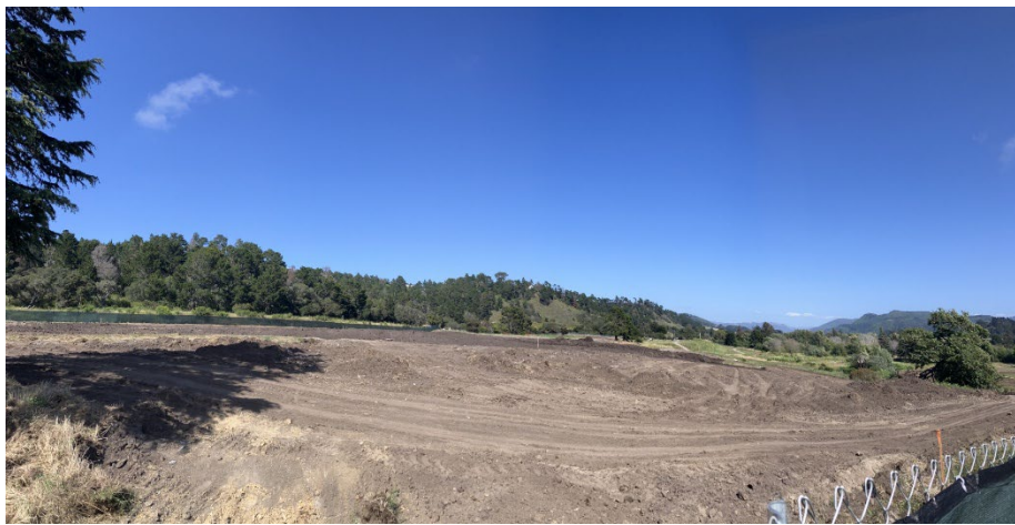
Photo 3: Construction staging area preparation activities.
