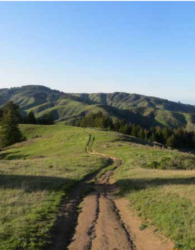
Erosion and rutting in the ridgeline roadways
