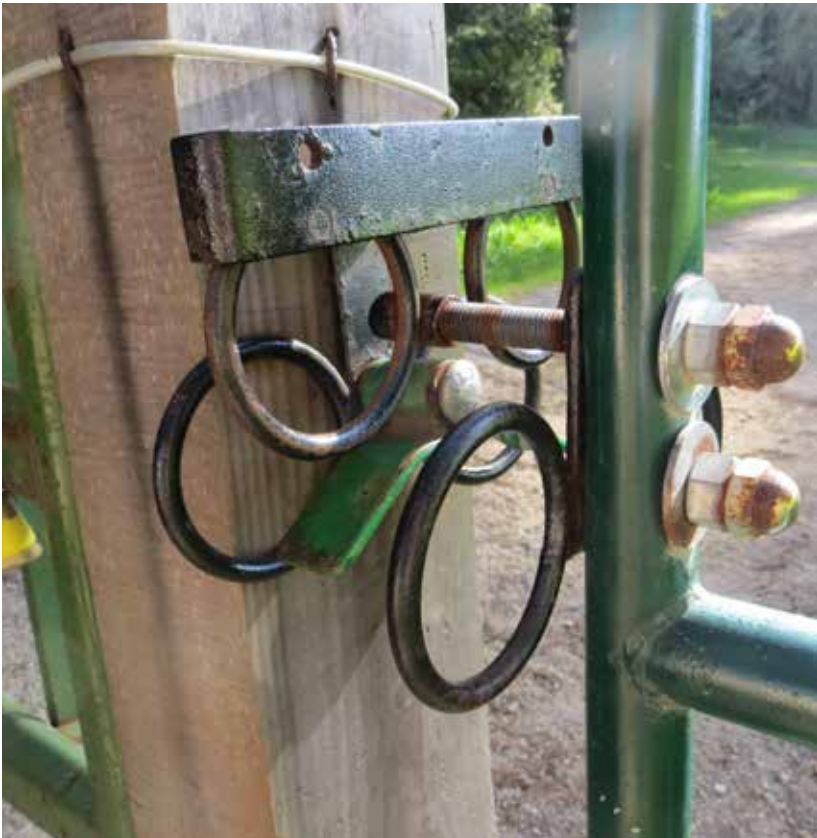
Double-ring gate closure allows gate to open in both directions
