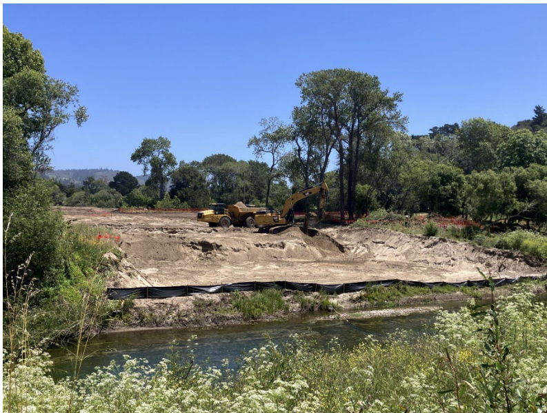
Photo 2: Rip Rap (large rocks armoring banks) being removed to prepare new temporary stream crossing for Phase 2.
