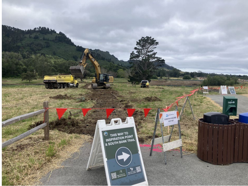
Photo 4: Removal of asphalt and concrete former cart paths near entrance plaza.
