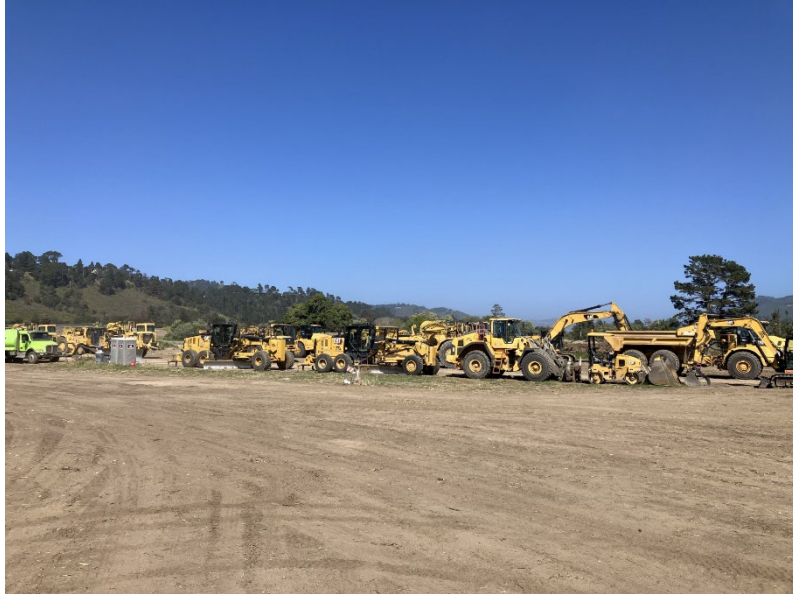
Photo 1: Contractor equipment mobilized and staged in the Park.
