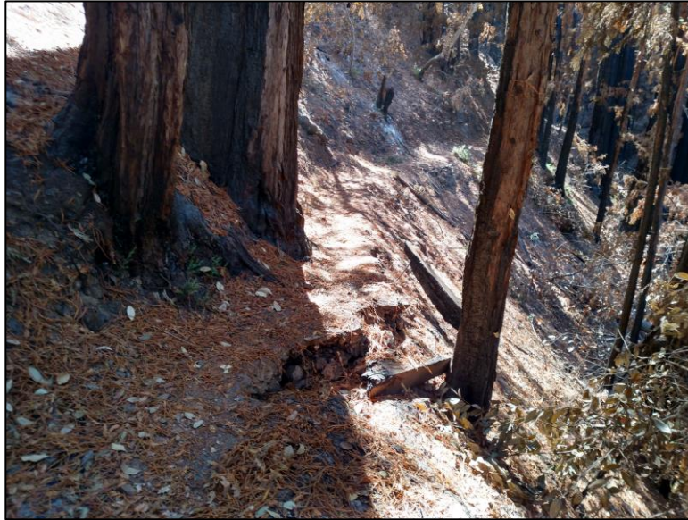
Figure 4: A retaining wall has completely burned and has left the trail dangerously undermined.
