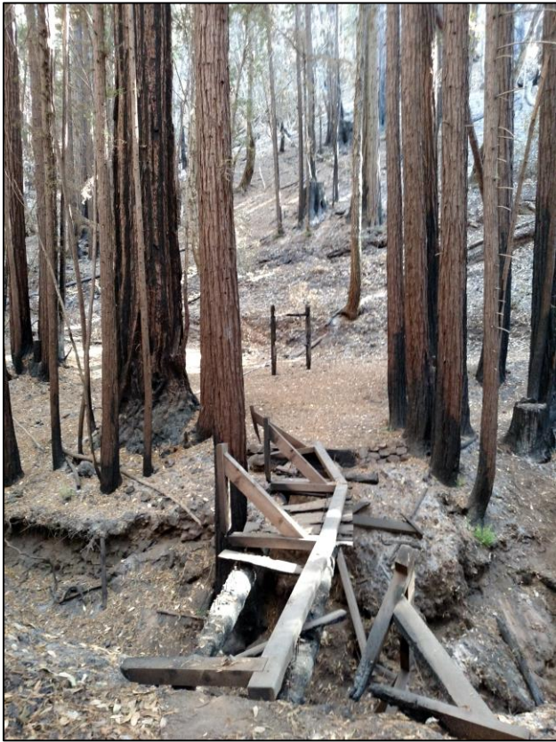
Figure 1: 27' bridge near the trailhead that needs a total replacement
