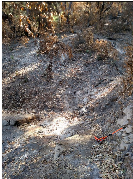
Figure 5: A puncheon burned here, but it was determined that due to the availability of local rock and the low flow this crossing gets that a armored drain crossing would be the most suitable structure at this location.
