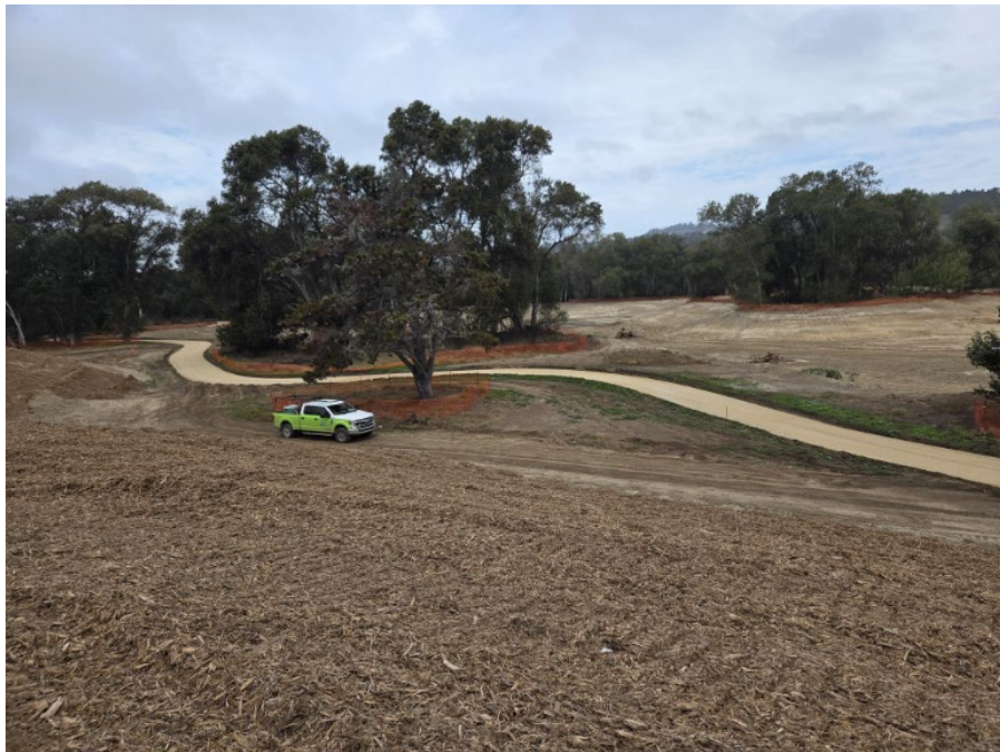
Photo 3: New aggregate trail segment constructed in the floodplain restoration area.
