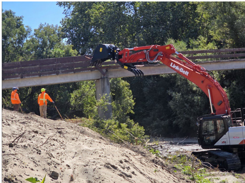
Photo 1: Looking at equipment beginning removal of former golf cart bridge (bridge 3).
