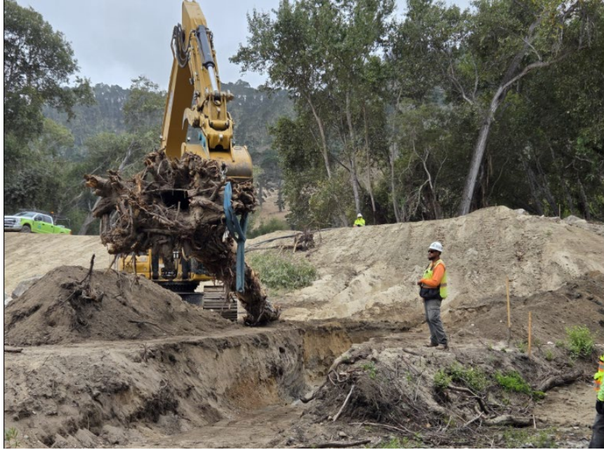
Photo 2: Installation of instream habitat structure (large woody debris) within the floodplain.
